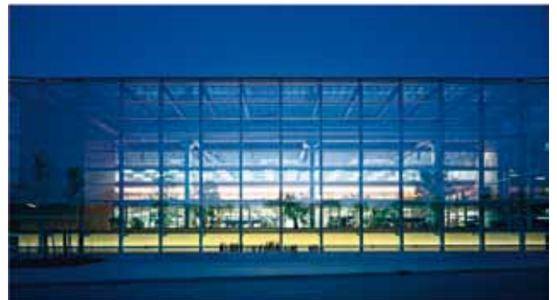
36 Service-Center von David Chipperfield
